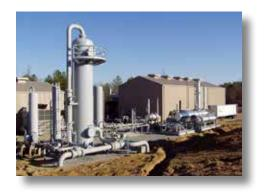
The MEG that returns from the well is termed Rich MEG and contains significant quantities of water, dissolved salts and other contaminants. **KASRAVAND** custom designs glycol regeneration systems to strip the absorbed water, salts, and contaminants from the Rich MEG to produce Lean MEG that can be recycled to storage tanks and production wells.
