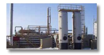
dehydration is the preferred technology over glycol dehydration. Certain applications, such as LNG processing, are suited to the use of solid desiccant adsorbents like molecular sieves and silica gels.
